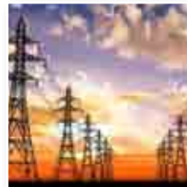
Utilities Power Generation
